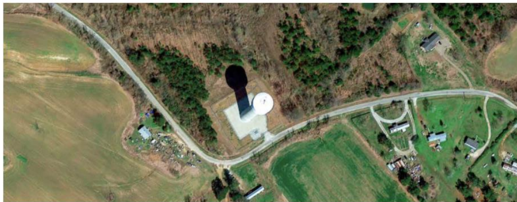
© Satellite image of a portion of the Megasite of West Tennessee. (Tennessee Department of General Services.)
