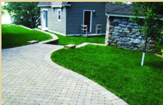
Figure 3: Pervious Paver System
