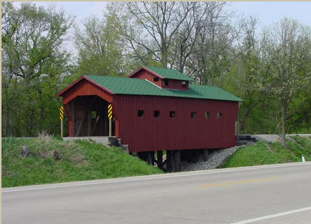
Figure 18: The covered bridge south of Fort Atkinson was built using boards from a nearby obsolete barn.
