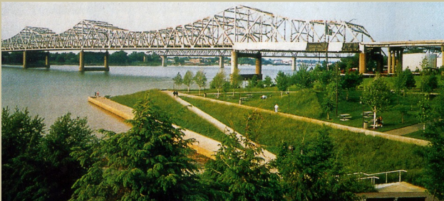
Figure 15: Bike and pedestrian trails provide a connection to the Mississippi River in La Crosse.
