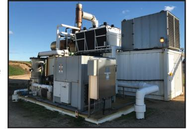
Electrical generation from methane produced by digester
