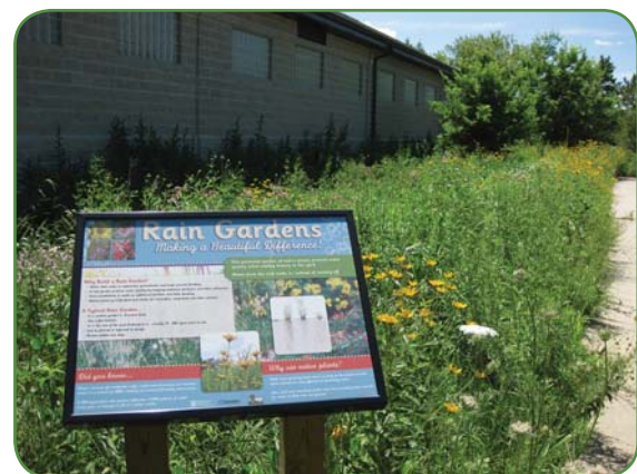
Rain garden and sign at Waukesha County's Naga-Waukee Maintenance Building
