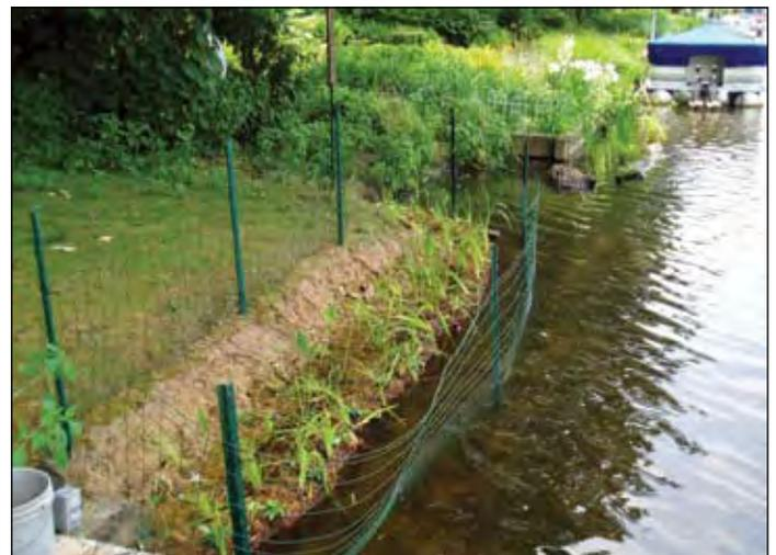
Figure 2. A re-established vegetated shoreline (l) and a newly installed and planted coir log (r).
