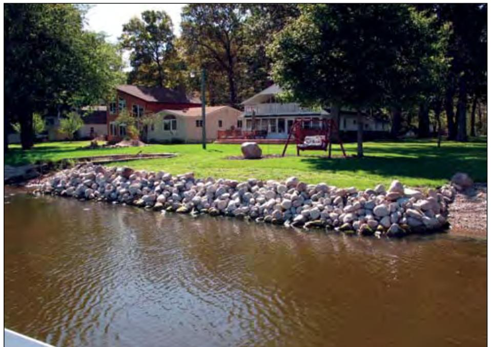
Figure 3. Glacial stone seawalls provide shoreline armoring while causing less damage to habitat and natural aesthetics.
