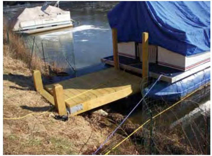
Figure 4. A recent compromise solution where “mini-docks” provide access over and adjacent to a shoreline re-vegetation project using coir logs.
