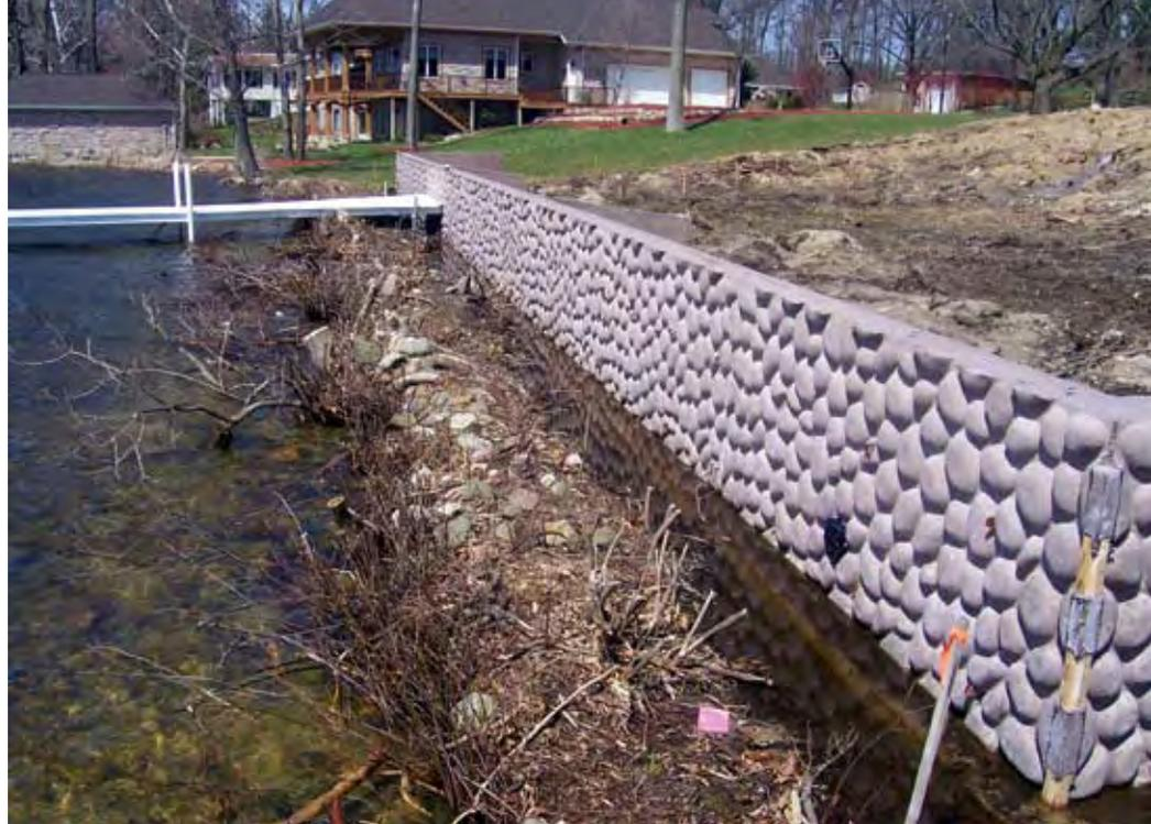
Figure 5. An example of a retaining wall installation.
