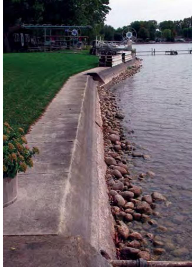
Figure 2. Bulkhead seawalls reflect wave energy and create barriers for many aquatic animals.
