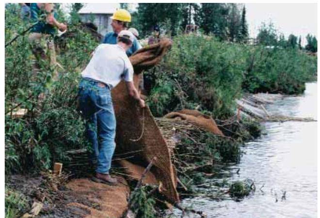
Second layer of a vegetated geogrid. Note first layer resting on top of tree revetment, Chena River, AK.
