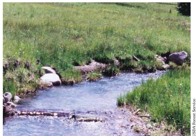
Coconut fiber log arresting bank toe erosion and becoming part of the bank.
