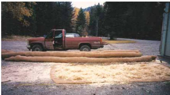
Constructing log using jute mat and hay with cuttings. Republic RD, Colville NF.
