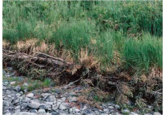
Small tree revetment stabilizing toe on Kenai River, AK. Note the healthy sedges.
