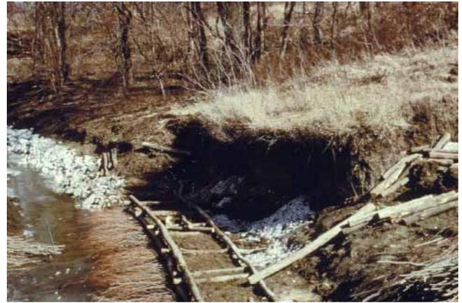
Live cribwall installation. Note live cuttings at bottom of photo and the next layer of frame on top of them.
