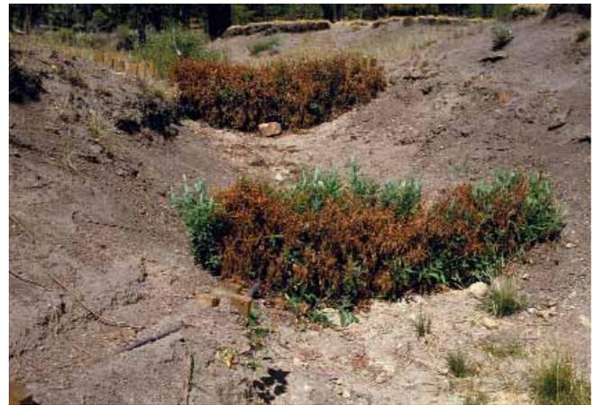
Trench packs in a gully with new spring growth. These were planted in the fall. They are approximately 1 in thick and 5 ft across. The cuttings are buried in 18 in of soil.
