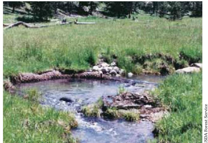
Coconut fiber log at bend in creek, protecting the toe of the bank. This log was placed into and across the creek to help create a pool for fish habitat.
