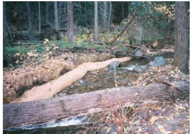
Note that the far end of this jute mat log is secured by rock, and the near end by a log. North Fork of O'Brien Creek, Republic RD, Colville NF.
