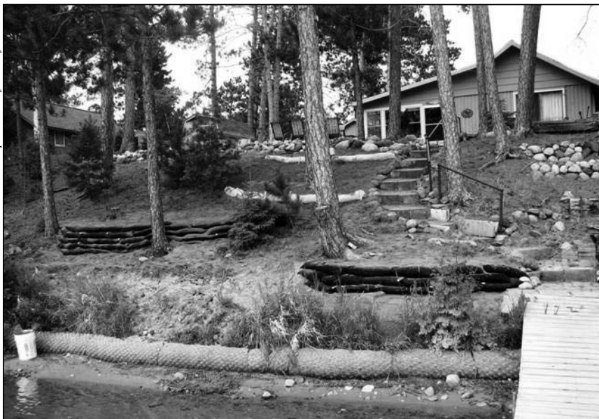
This view of a property on Found Lake in Vilas County shows the use of EnviroLok bags™, biologs and native plants.
