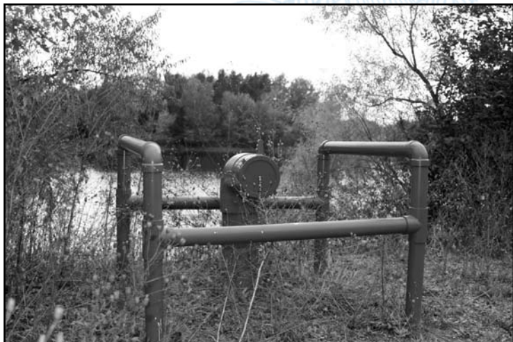
A dry hydrant is a non-pressurized pipe installed at a water body that is in close proximity to an all weather road.
