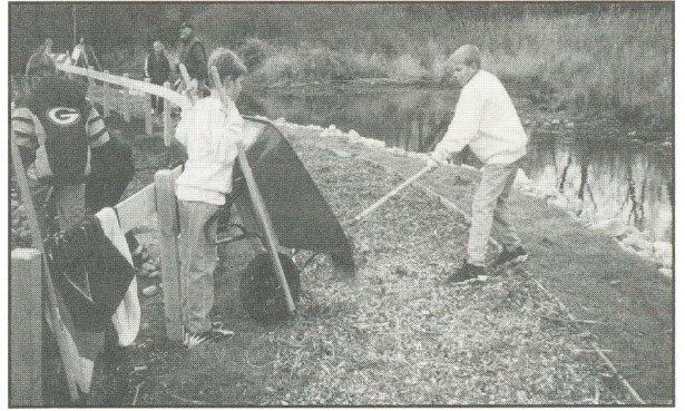
Students constructed fences, placed riprap, laid sod, and are now adding bark chips to finish the trail along the Pewaukee River.
