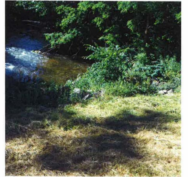
Right Side, Downstream Embankment
