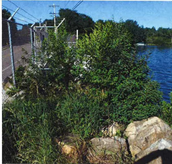
Right Side, Upstream Embankment
