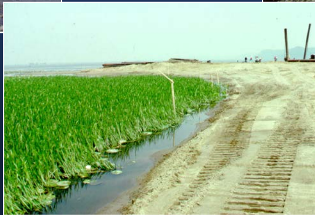
Sand base and work limit stake
