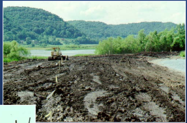
Shaping fine material (topsoil)
