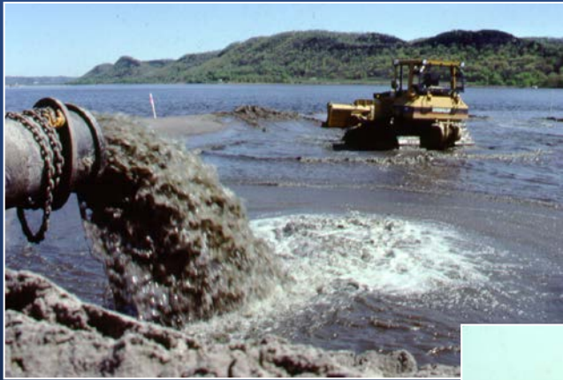
Constructing sand base with dredged material
