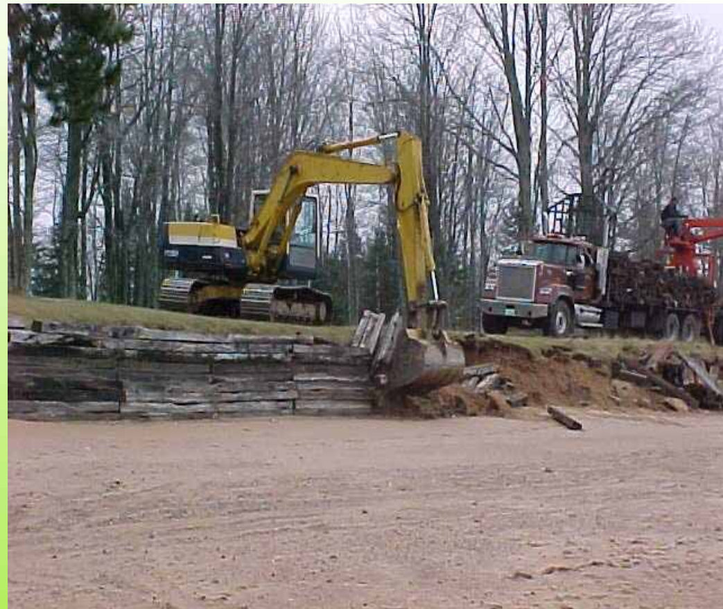
Seawall Removal
