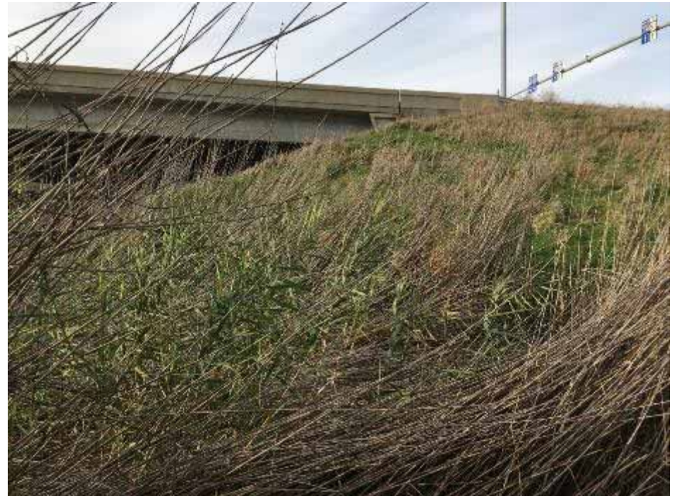
Landmarks in the background help orient the picture.
