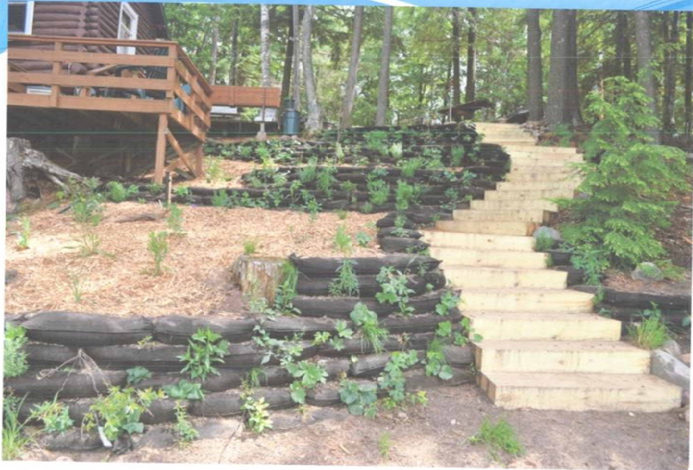
Vegetated Retaining Walls - Geotextile Bags (Install)
