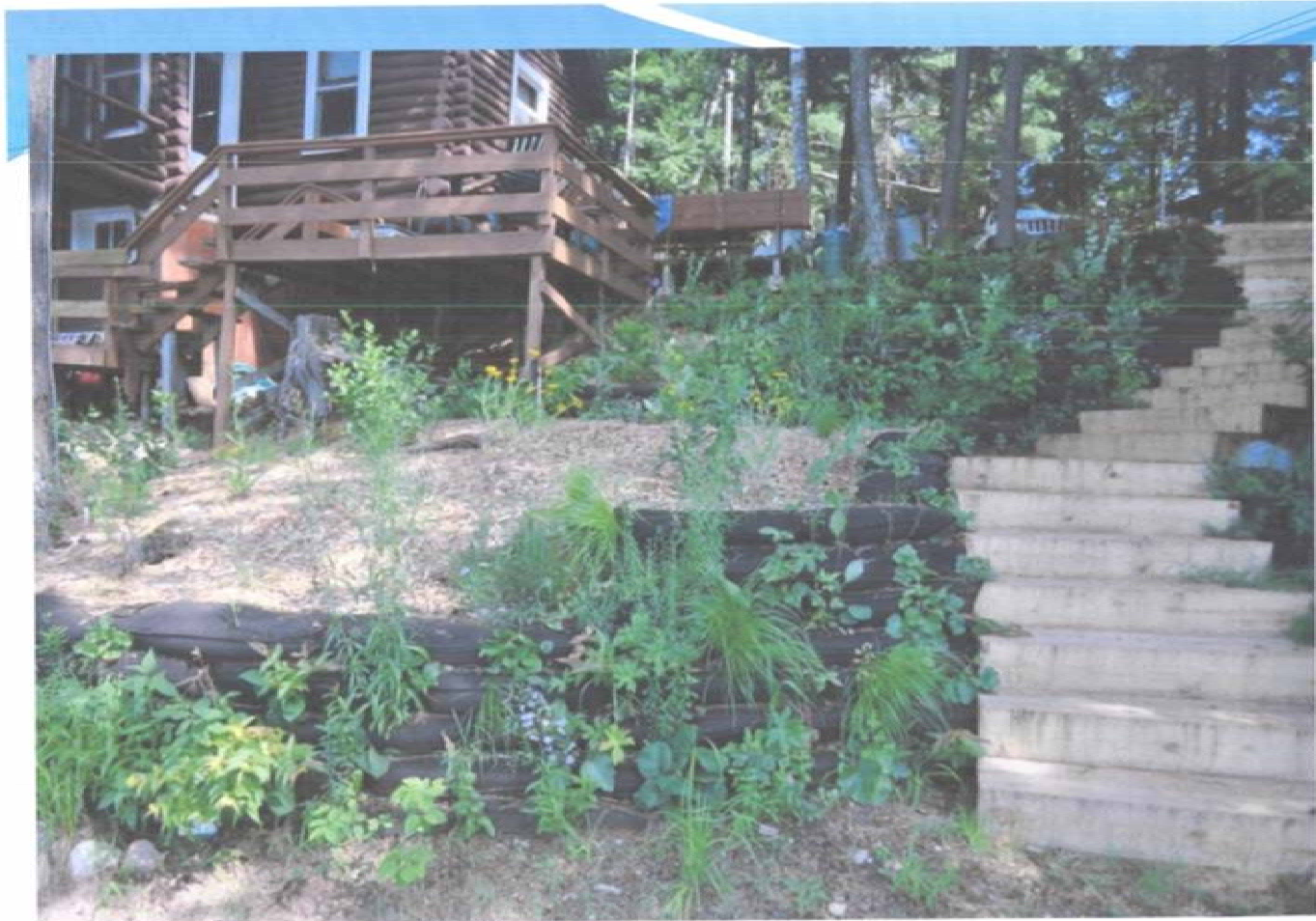
Vegetated Retaining Walls - Geotextile Bags (After)
