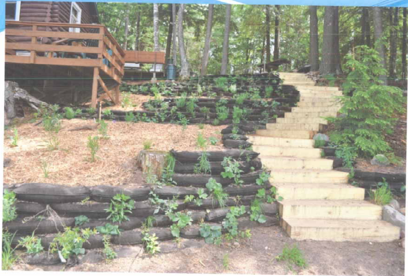
Vegetated Retaining Walls - Geotextile Bags (Install)
