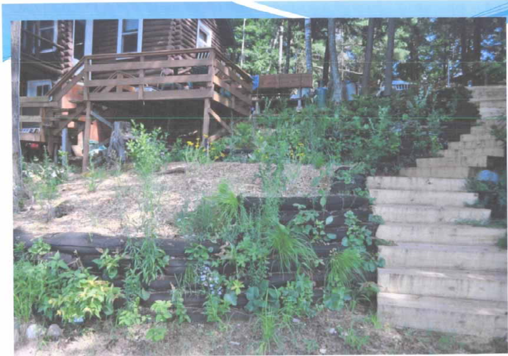
Vegetated Retaining Walls - Geotextile Bags (After)
