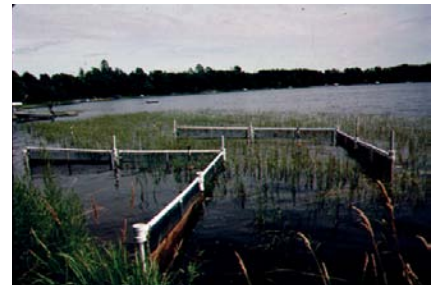
Figure 2. An effective wave break design provides protection from wave impacts to newly planted aquatic and transition zone vegetation during establishment. Transition and aquatic zone vegetation is planted in the sheltered area within each "V." Wave breaks are used until plants are well established, sometimes up to three or four years. They must be removed in autumn before lakes freeze and reinstalled the following spring after ice thaw.
