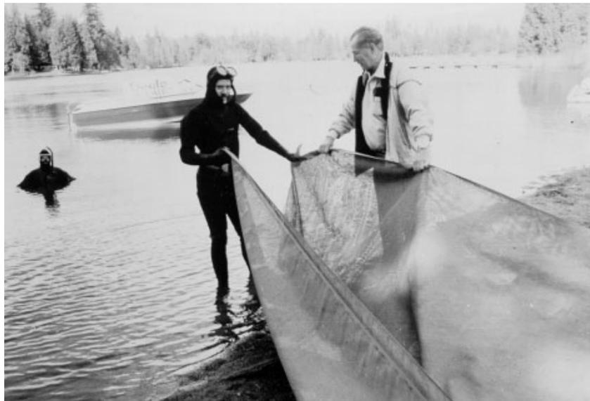
A fiberglass screen, weighted with rebar, being set by divers on the bottom of Pipe Lake, King County, Washington.
