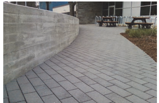
A concrete paver walkway in Burlington.
