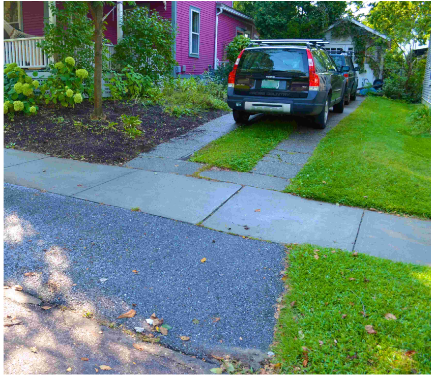
A ribbon or "Hollywood" driveway, like this one in Burlington, is another stormwater-friendly driveway option.
