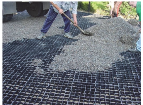
Installation of a plastic grid system with gravel fill (groundprotection.co.uk)
