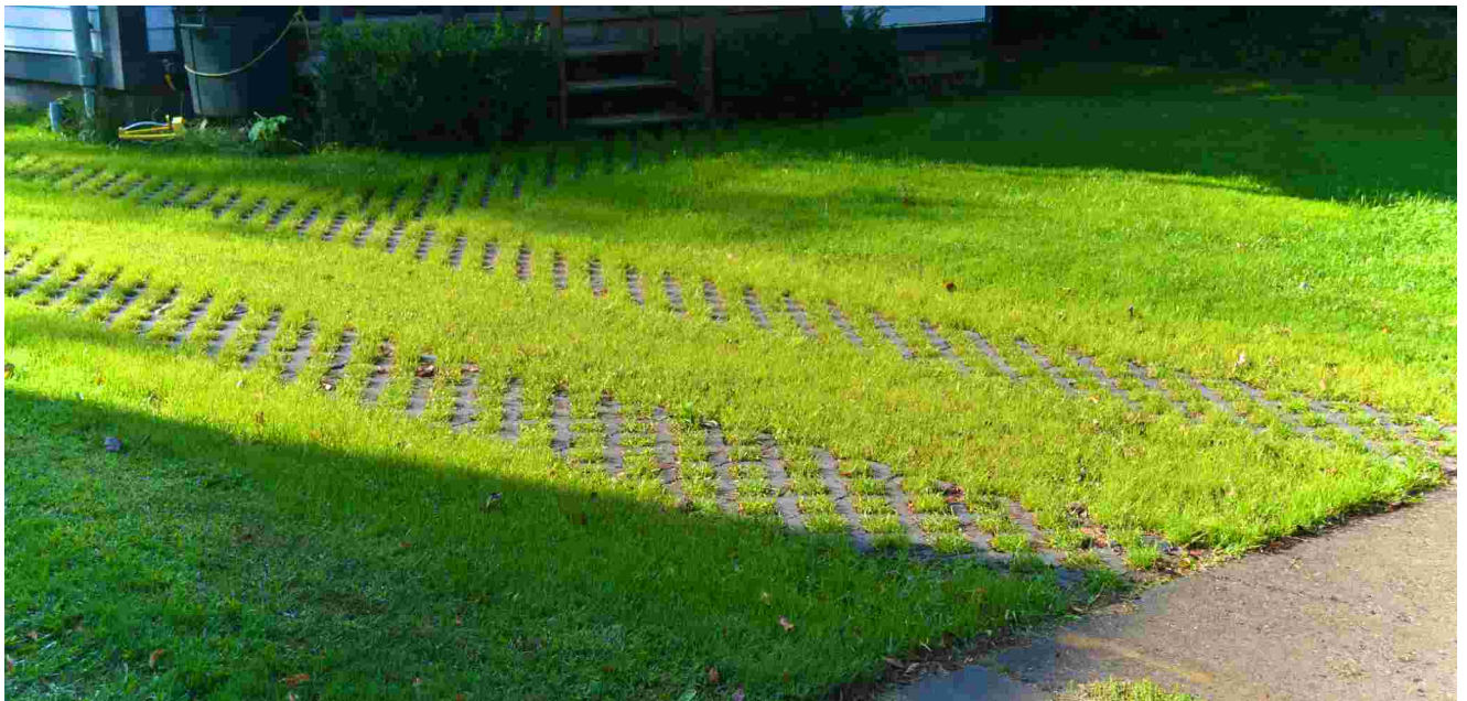
Stormwater friendly driveways like this one in Burlington, where an open concrete paver system was planted with grass, offer multiple benefits for homeowners, local infrastructure, and Lake Champlain.
