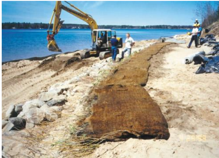
Installing the pre-grown brush layer mats in the vegetated geogrid.
