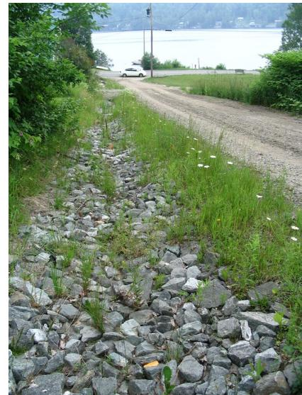
At left, lake association members seed and mulched a newly cleaned ditch. Center, rip rap stabilizes a culvert inlet area, often a site of either road edge erosion, or inlet pool erosion. At right, a steep road that serves several camps has had a rock lined installed to prevent the previously on-going erosion of the ditch.
