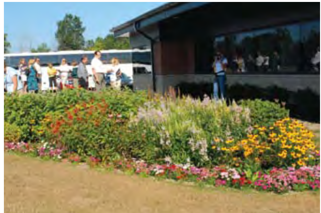
Bioretention is one variation of an infiltration BMP, such as this rain garden at the Macomb County Public Works Building
