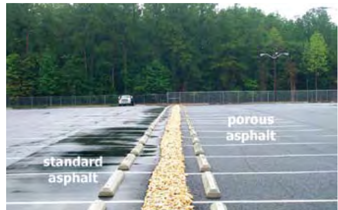
Figure 7.33 Riverstone edge serves as a backup inlet into the infiltration bed under the porous asphalt
