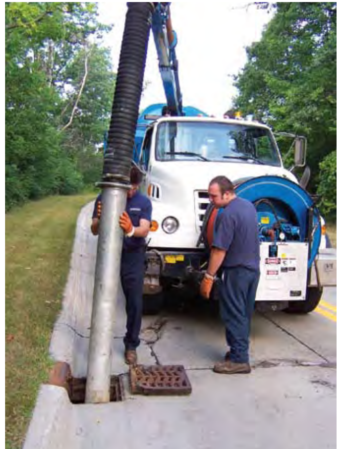
Catch basin cleaning in Bloomfield Township, MI
