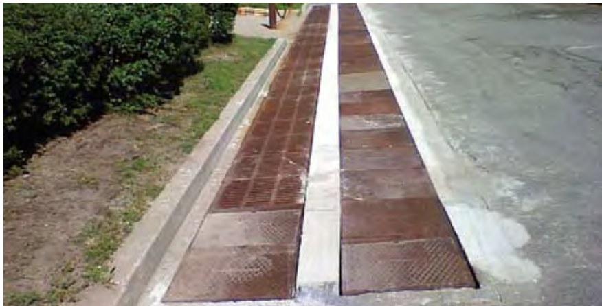
Sand filter in the City of Wayne, MI
