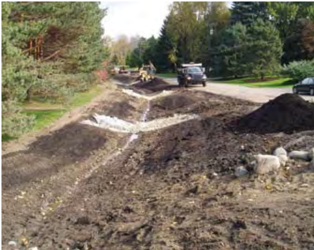
Construction of Meadowlake Farms bioswale with infiltration, Bloomfield Township, MI.
