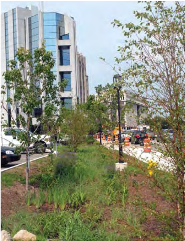
Bioswale at Macomb County Administration Building, Mt. Clemens, MI.
