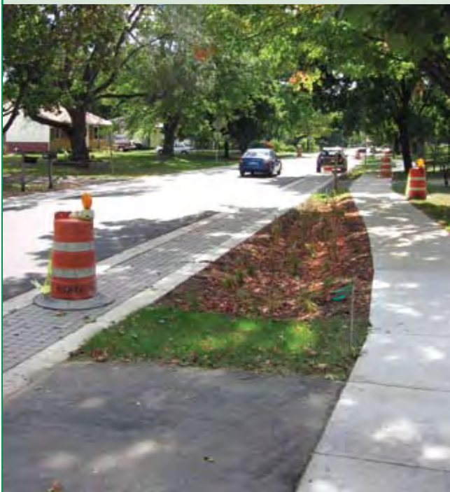
East Street reconstruction consisting of 26-foot asphalt section converted to 18 feet of asphalt with two 3.5-foot concrete porous paver strips (and ribbon curb) that infiltrates all road runoff and some rooftop and sidewalk runoff.
