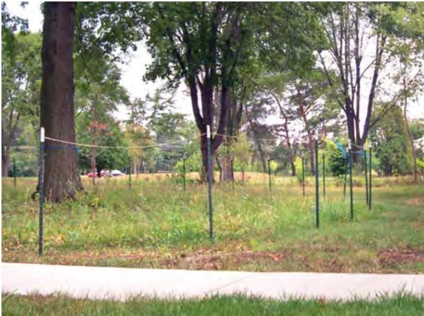
Fencing around oak tree to minimize soil compaction
