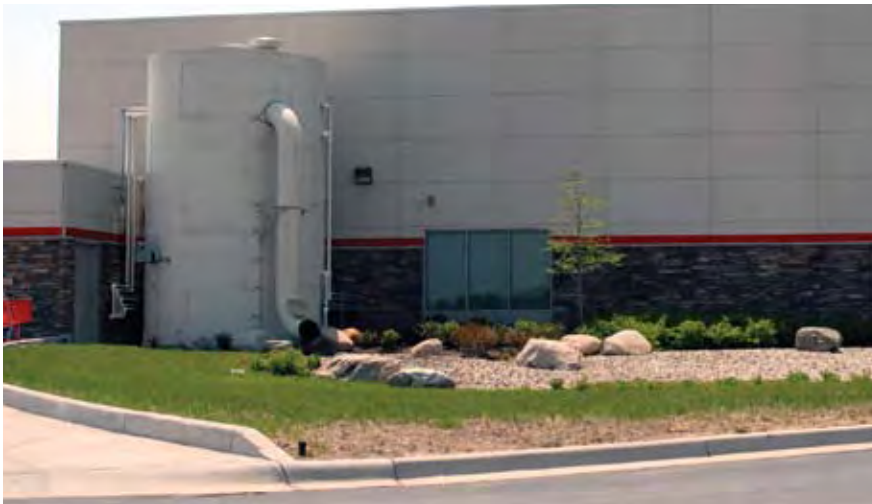
Cistern at Fairlane Green shopping center, Allen Park, MI
