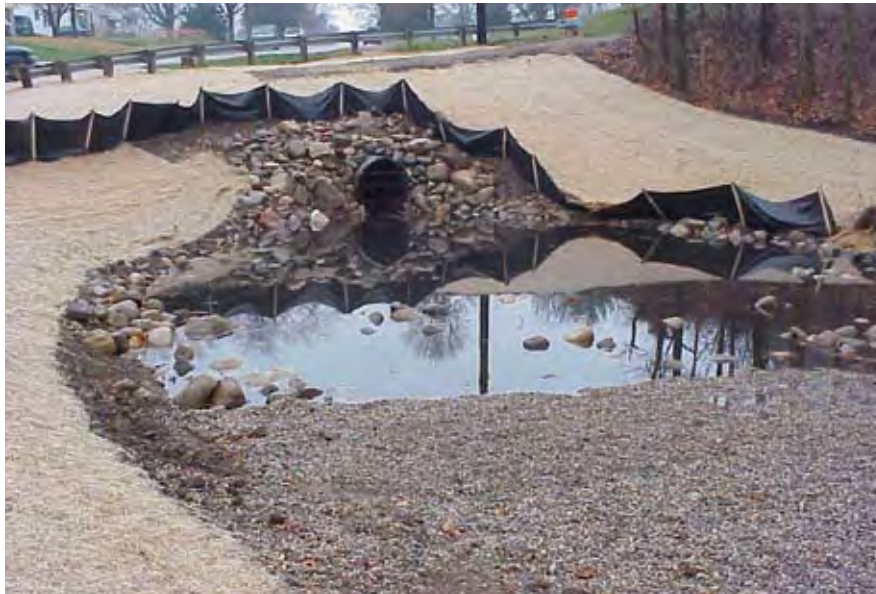
LaVista Storm Drain Project Level Spreader Source: City of Battle Creek
