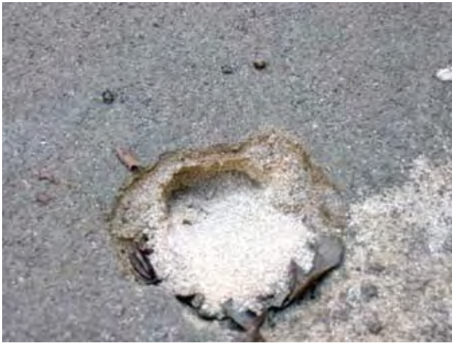
A discolored film on top of a sand filter indicates the need for maintenance
