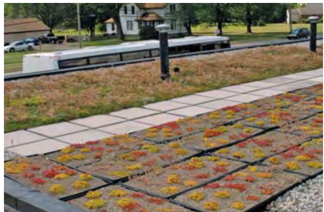
Frasier School District is testing both the tray system (foreground) and mat system (background) on their operations and maintenance building.
