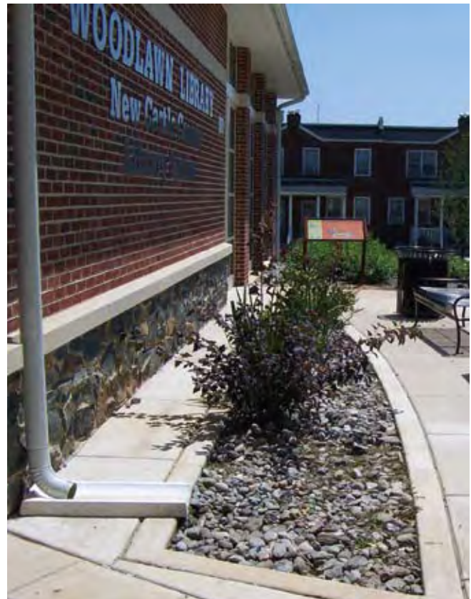
Example of Infiltration Planter Box
