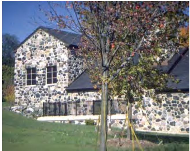
CSO Retention Treatment Basin in the City of Birmingham Source: Rouge River National Wet Weather Demonstration Project.
