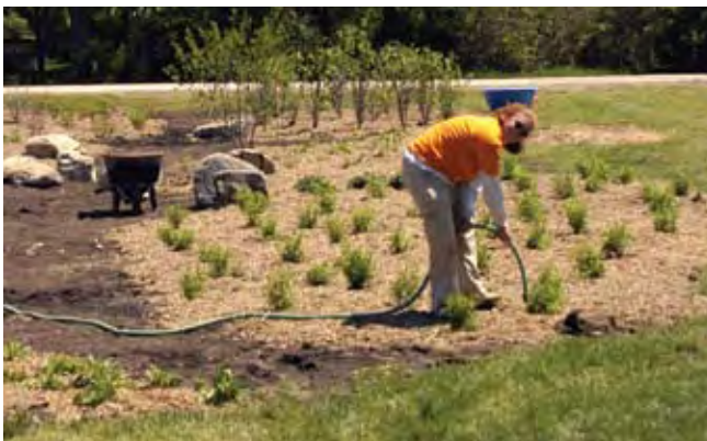
Watering newly established vegetation
