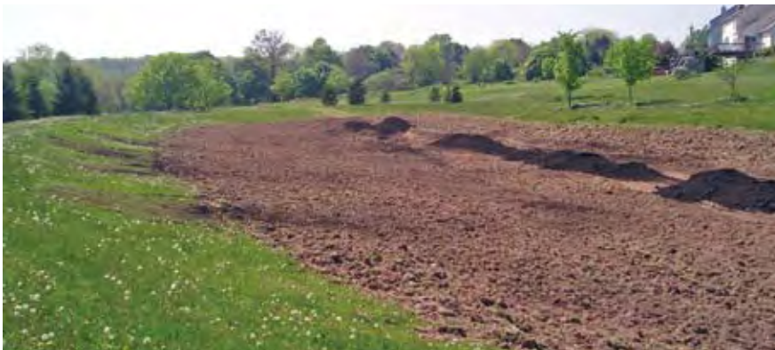
The soil in the detention basin pictured above was amended with compost.
