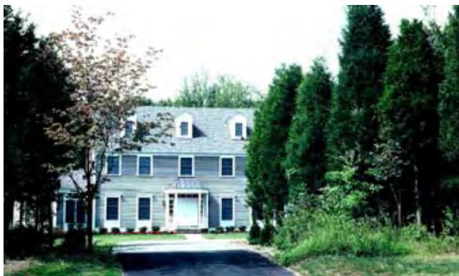
Disturbance of native trees minimized during residential construction
