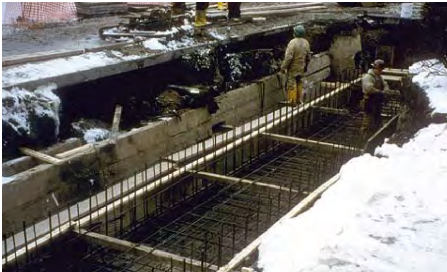
Installation of a sand filter
