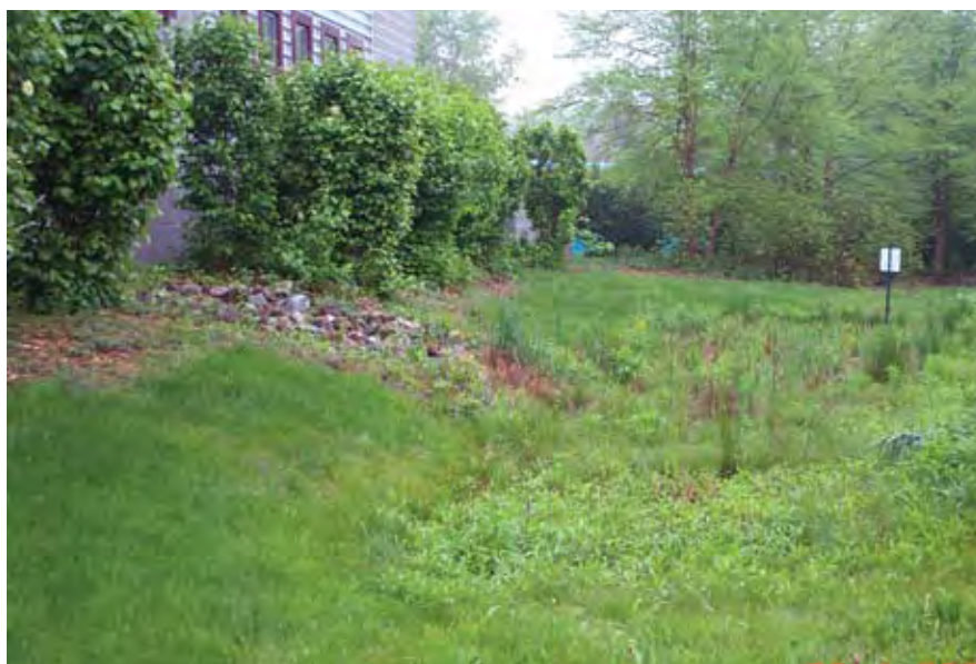
Roofleader directed toward bioretention
