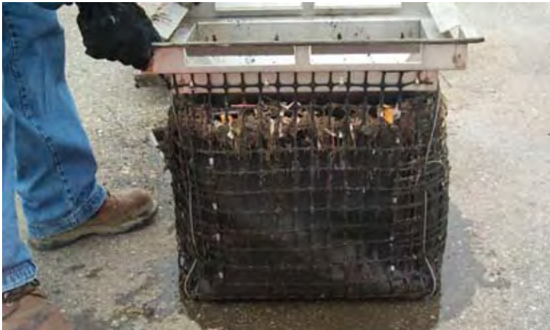
Filtration insert with debris in St. Clair Shores, MI
