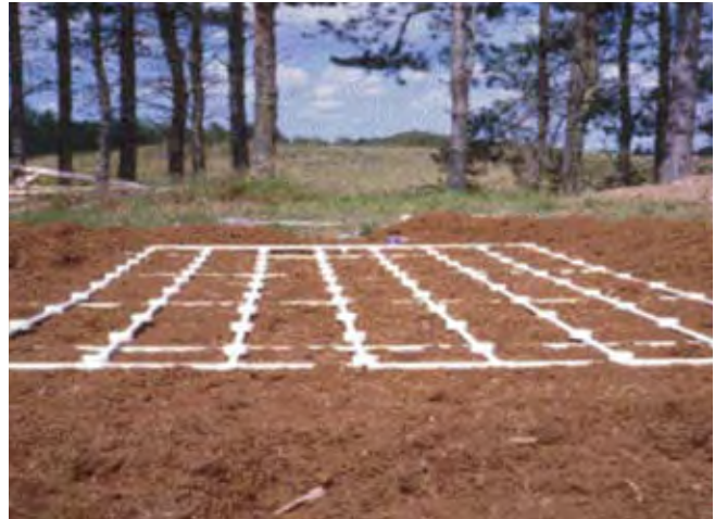
Placement of a pipe distribution network in a peat filter
