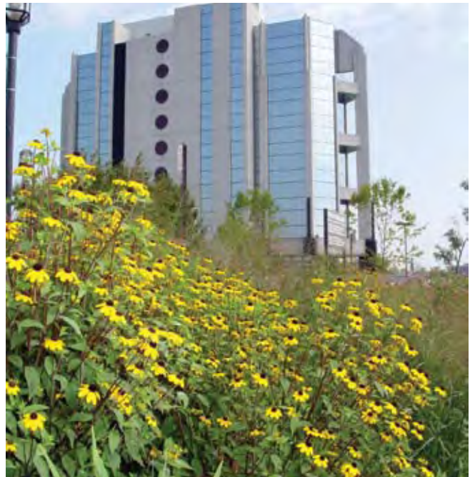
Rain garden at Macomb County building in Mt. Clemens, MI
