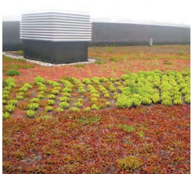
Vegetated Roof at Lawrence Technological University
