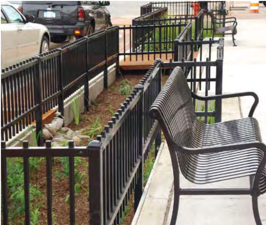
Michigan Avenue bioretention planter box
