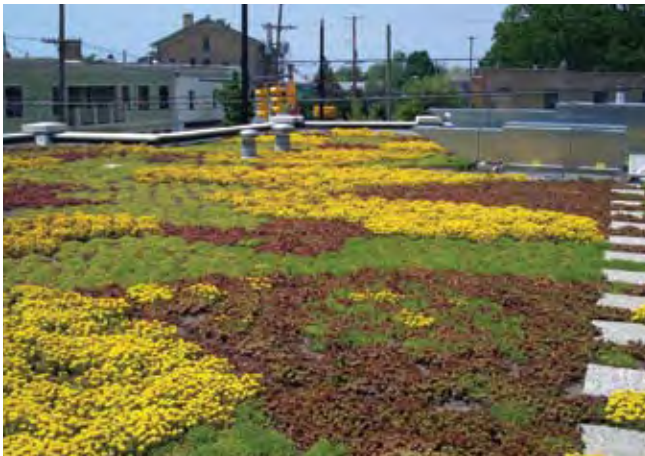
Vegetated roof on East Hills Center
