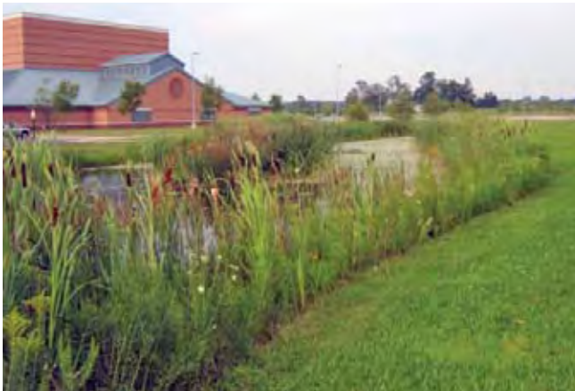
Constructed wetland at Okemos High School
