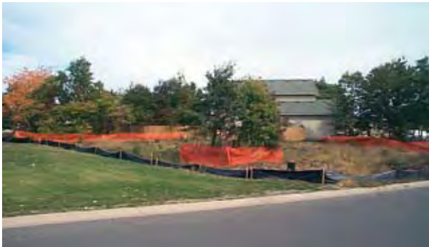
Preventing soil compaction adjacent to a stand of trees Source: City of Andover, Minnesota
