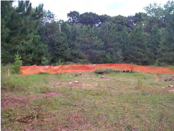
Minimizing disturbance of soil to protect wooded area Source: City of Andover, Minnesota
