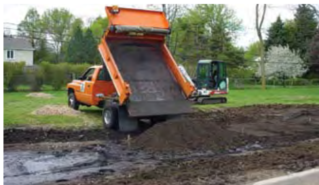
Preparing bed with planting soil
