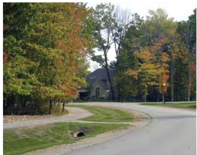
Stormwater disconnection in Washington Township, MI
