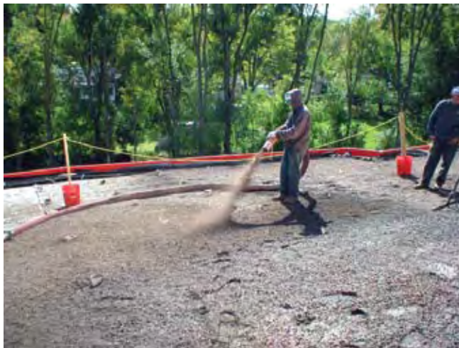
Blowing media onto Mallet’s Creek Library Roof, Ann Arbor, MI
