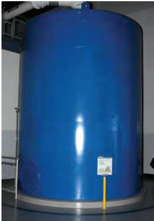
Ford Rouge Plant cistern
