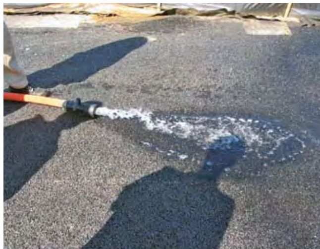
Figure 7.41 Testing permeability with a high capacity hose
