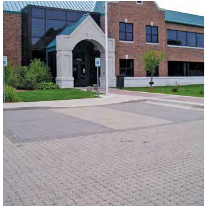
Permeable paver lot at Grand Rapids Environmental Services Building
