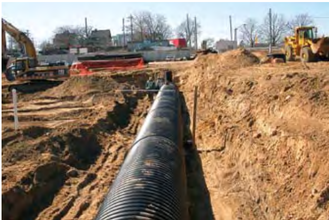
Subsurface infiltration system
