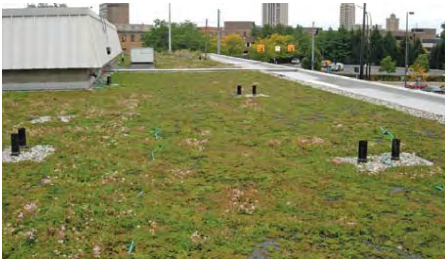
Green roof on City of Battle Creek Police Department building Source: City of Battle Creek
