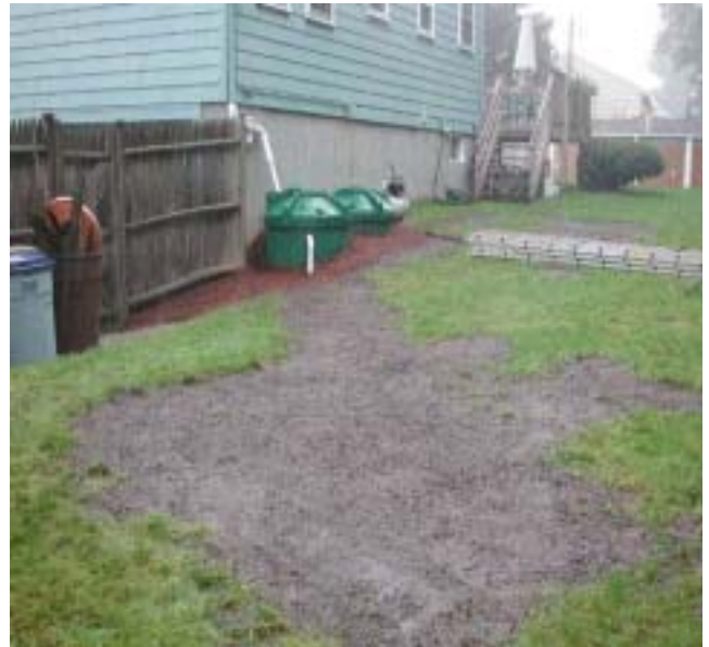
Manufactured dry well system after installation. The dirt areas indicate where the well was buried. The green objects are storage tanks with a pump. Drywells also work well receiving rain barrel overflow (Photo: Charles River Watershed Association)
