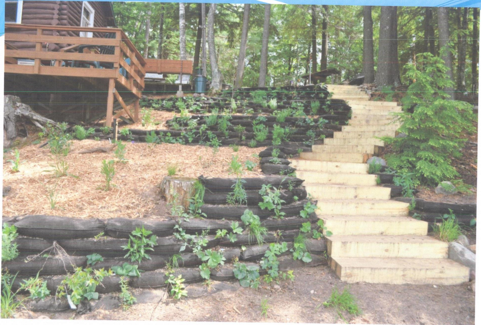
Vegetated Retaining Walls - Geotextile Bags (Install)
