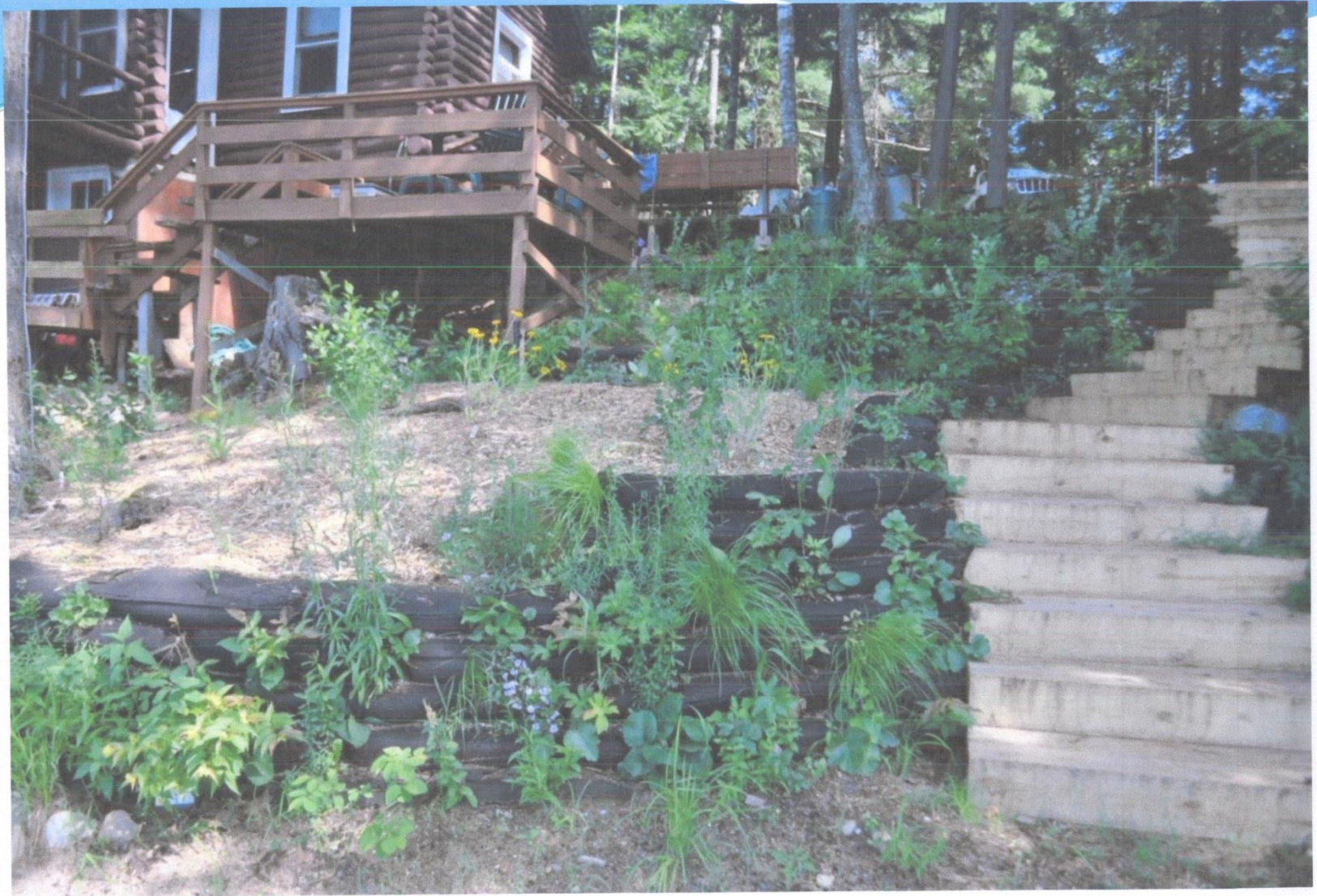
Vegetated Retaining Walls - Geotextile Bags (After)
