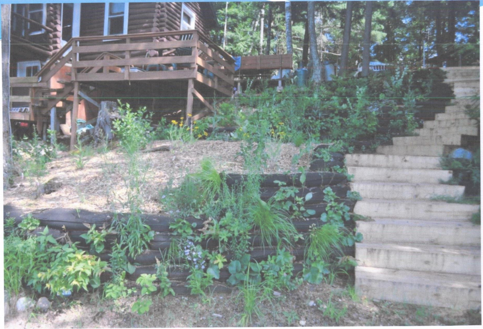
Vegetated Retaining Walls - Geotextile Bags (After)
