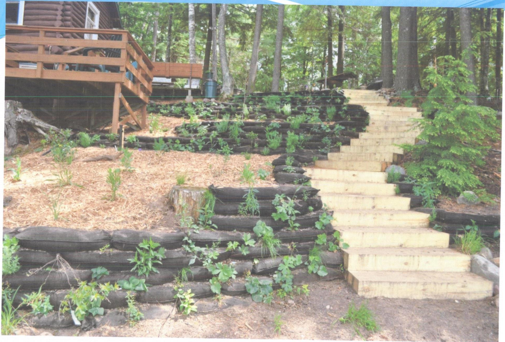
Vegetated Retaining Walls - Geotextile Bags (Install)
