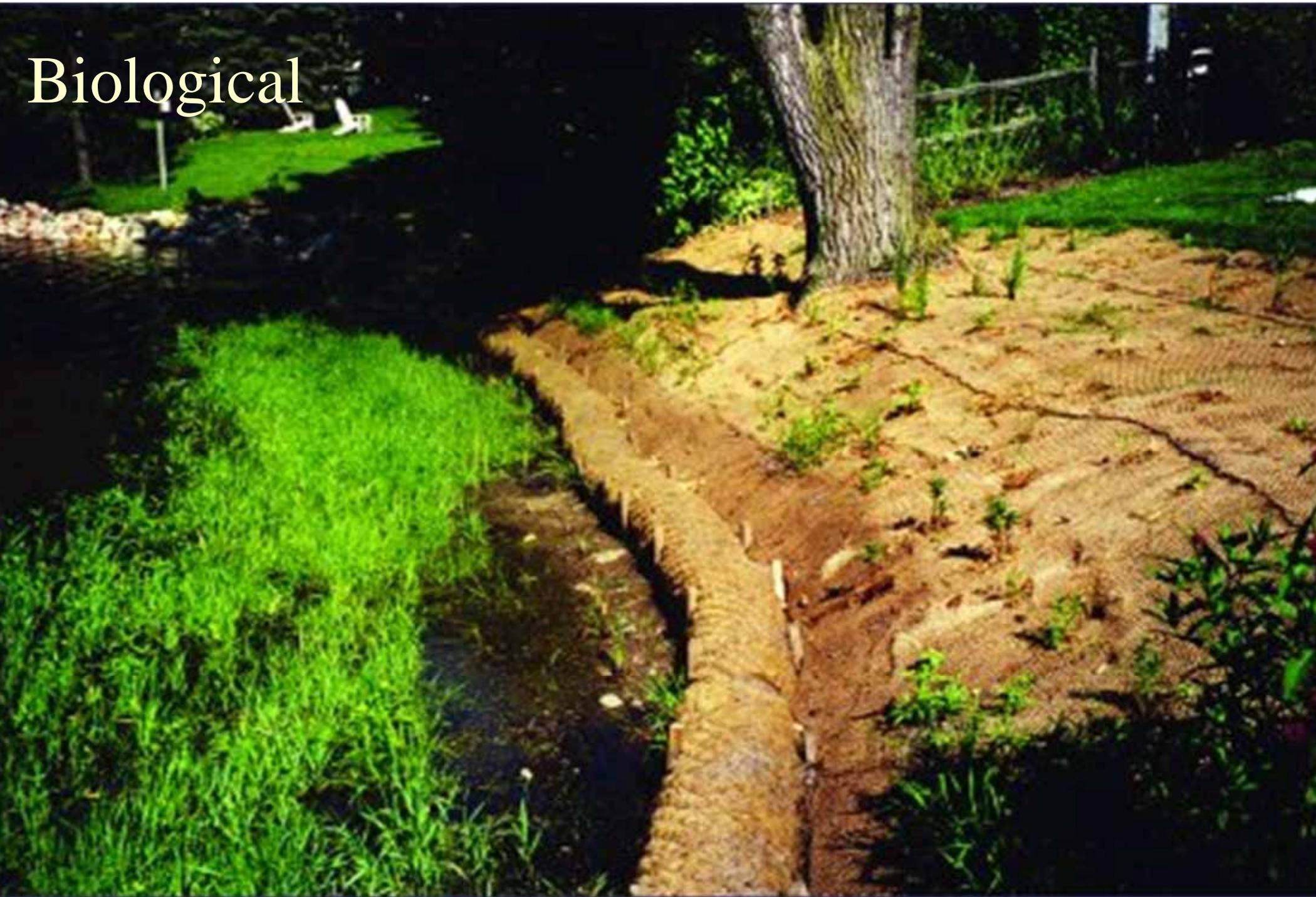
**Figure 16-36** Coconut fiber roll details
