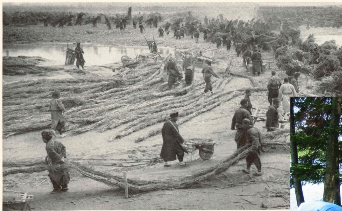
Swarming Along the River Bank Like Ants, Coolies Drag Long Strands of Woven Willow Sticks to the water's edge. Others carry packs of kaoliang stalks to the water's edge. Both materials rot in the water after a few years. Then new stacks are placed on top of the decayed mass into the mud on the river bottom. Often the entire construction is destroyed when the current scours out the river bed.
