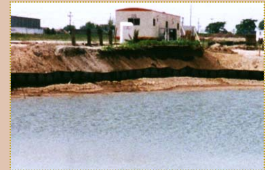
Construction site in summer of 1999.
