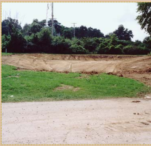
Infiltration trench during construction and seeding.
