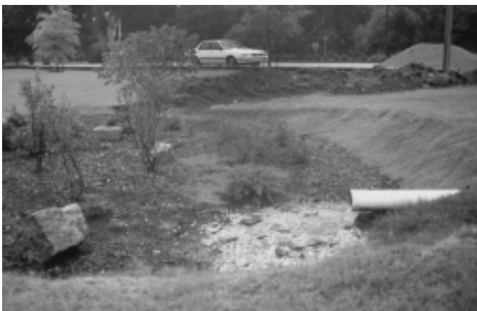
Figure 1. Rain garden installed at Neuseway Nature Center (Kinston, N.C.). Stormwater runoff enters through the 6-inch-diameter pipe near the right foreground. The garden receives rainfall from a nearby rooftop. This rain garden is a small depression in sandy soil. The mulch is hardwood.
