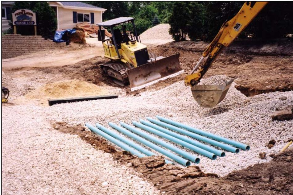
Example of a co-operator at a commercial site utilizing a subsurface retention system to collect and treat stormwater runoff thereby improving the quality and reducing the quantity of runoff entering Pike Lake.
