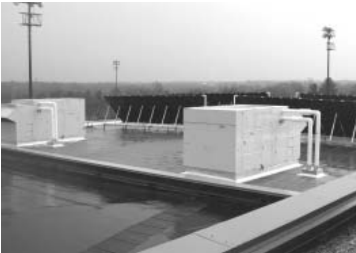
(top) The James Madison Memorial High School in Madison, Wisconsin worked with the MGE Foundation to install this 2.4 kW solar electric system over the south entrance of the building.
