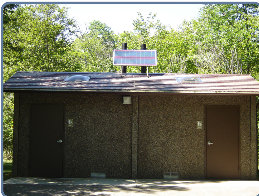
This solar electric panel provides lights for a restroom at Cave Point County Park in Door County, WI. The building has very energy-efficient lights to conserve energy, thus reducing the amount of solar panel needed.
