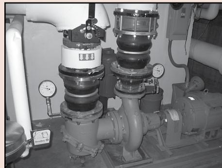
This pump circulates hot water from the boiler room to various parts of the school building.
