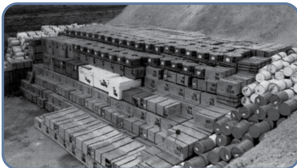
Solid low-level waste is safely disposed of in shallow trenches. When the trench is full, a protective covering for erosion control will be placed on top. Source: U.S. Department of Energy
